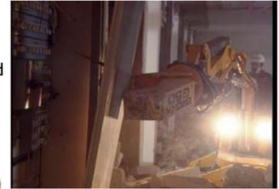
The G50 is the ideal tool for soft demolition such as removal of dry walls, piping, ventilation ducts and even sorting of material on site.
