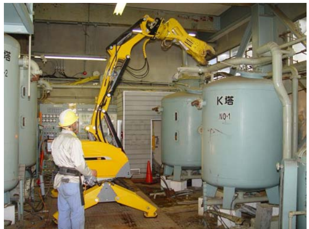
Brokk 180 with steel shear at the Water Treatment Plant
