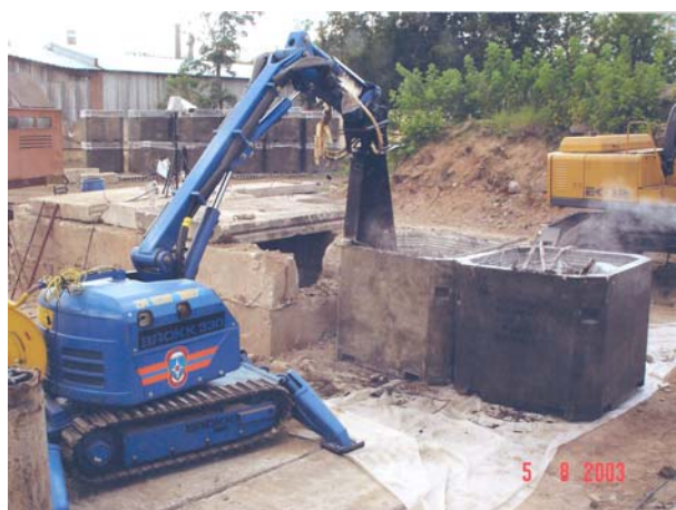
Brokk 330 with steel shear
