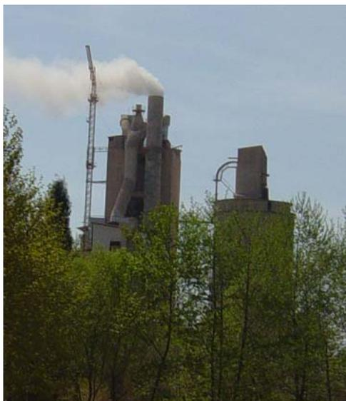
The 70 metre kiln at Neka Cement has a diameter of 4.65 m. The plant calculates with three downtime periods a year for kiln maintenance, during which time valuable production is lost. To shorten the downtime periods is thus of major importance to the profitability of the plant.
